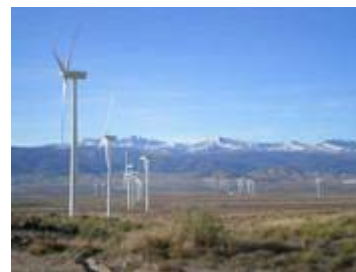
Spain El Marquesado Wind Farm, Granada, with installed capacity: 198 MW.
