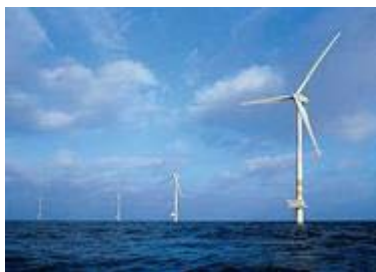
Germany Windpark Butendiek, Hamburg, with installed capacity: 240 MW.
