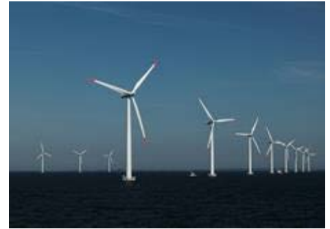
An offshore wind farm located at Rodsand of Denmark, with 72 wind turbines, total installed capacity of 165.6 MW.
