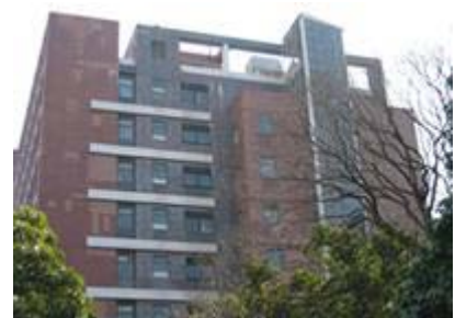
PV panels mounted on Chow Yei Ching Building, HKU.
