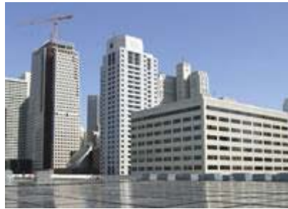
Courtesy: IEA PVPS website: http:// www.iea-pvps.org Copyright: PowerLight Corp.
