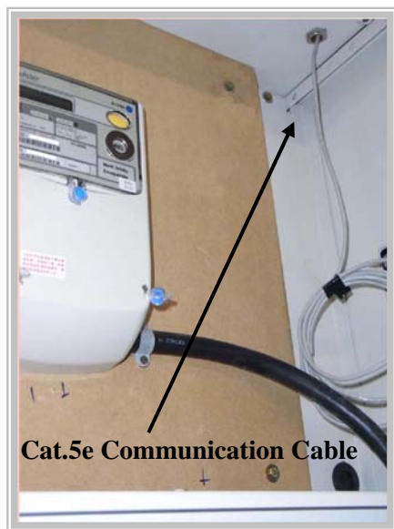
Figure 8 – Cat. 5e Communication Cable
