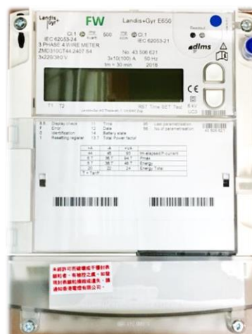
Three Phase RE Meter
