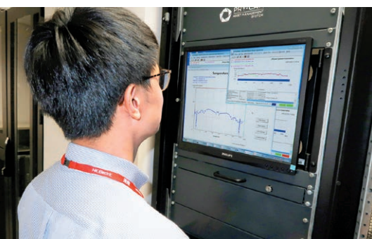
On-line monitoring of temperature distribution of a transmission cable section 利用在線系統監察電纜溫度的分佈
