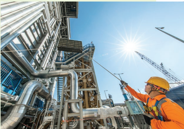
Selective Catalytic Reduction Systems under installation
