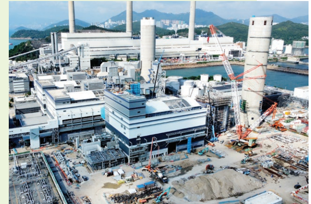
Gas-fired generating unit L12 under construction
