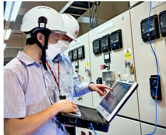
The monitoring system is installed above the switchgear panel
