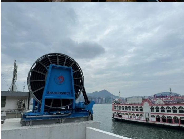
HK Electric supports the installation of charging infrastructure at North Point Ferry Pier (blue equipment shown in the photo).
