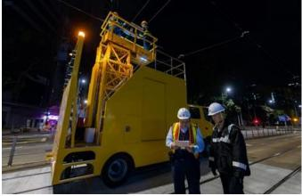
HK Tramways deploys an engineering vehicle equipped with an elevating work platform to switch over the power supply to another one and resume tram services. HK Electric engineers provide support on site.
