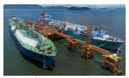
The Hong Kong offshore LNG terminal, jointly developed and constructed by CLP Power and HK Electric, has gone into service. The photos show the first LNG shipment under a long-term supply agreement arriving at the terminal. The shipment (left) was unloaded to the Floating Storage and Regasification Unit (FSRU) vessel (right) before it is sent to CLP Power's Black Point Power Station and HK Electric's Lamma Power Station through two separate undersea pipelines.
