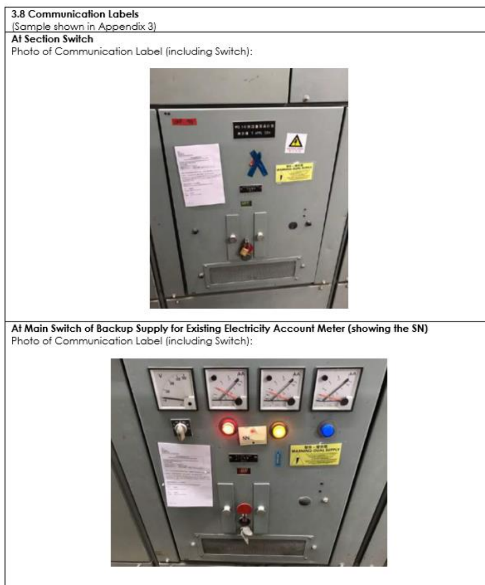
Figure 5 – Sample of Photos for Communication Labels at Section Switch and/or Main Switch of Backup Supply for Existing Electricity Account Meter
